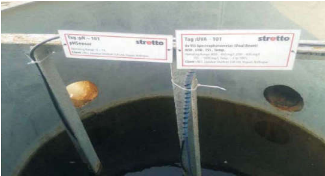
Sensor for outlet Treated Water -for parameter pH, T.S.S, C.O.D & BOD measurement.
