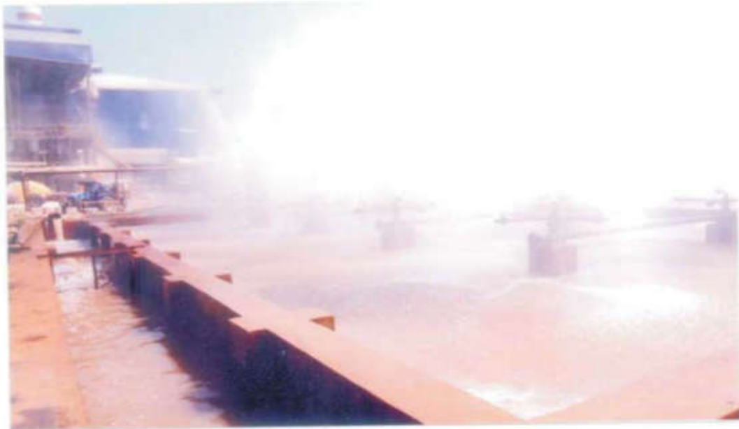
Mini spray pond capacity 10200 M 3 /day water recycle inlet temperature 58°C to 60°C outlet temperature 28 to 30°C
