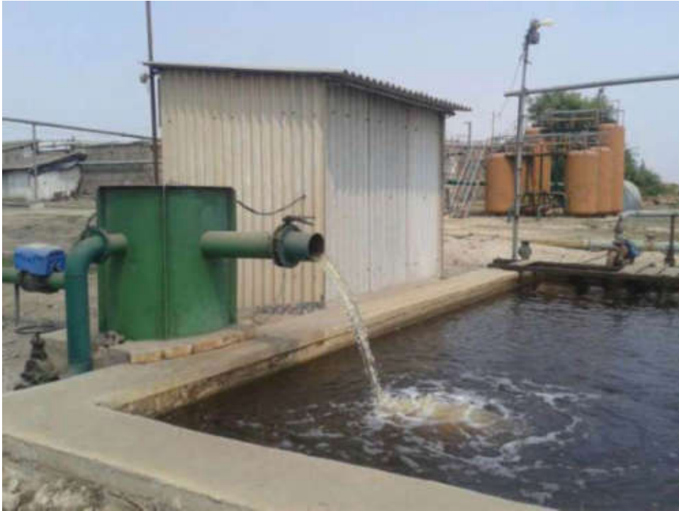
Treated Water Outlet
