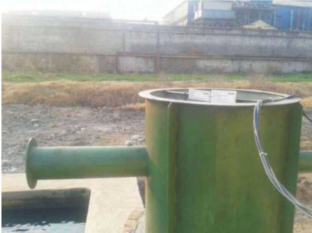
Treated Water outlet Tank
