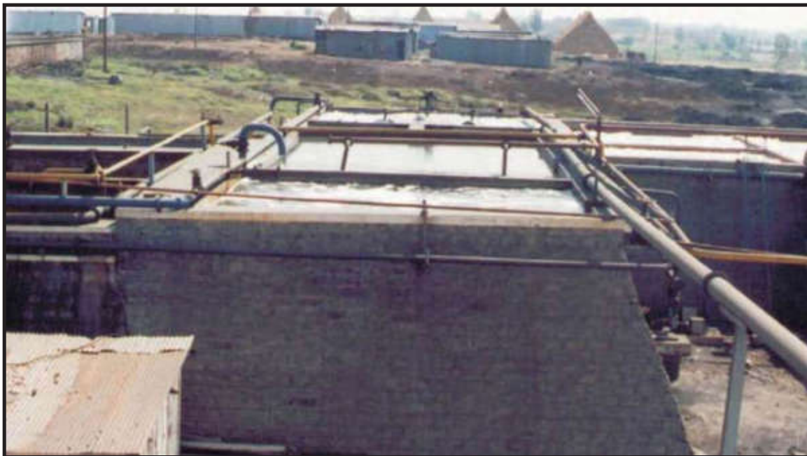
Floating areator, sludge seperator & return sludge to digester & preareation tank
