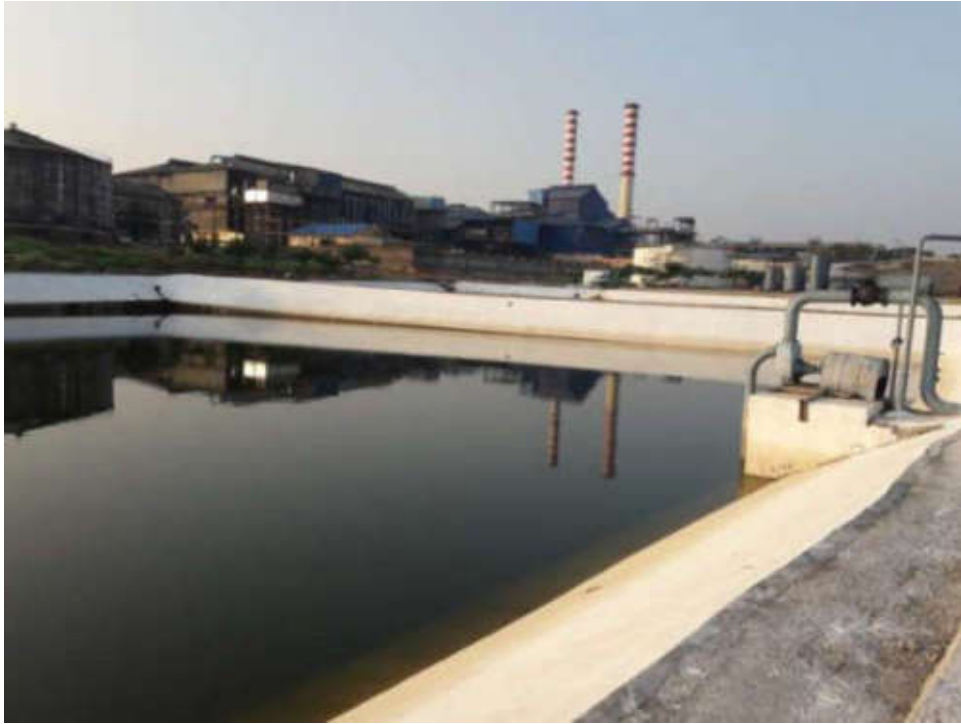
15 Days Storage Tank-1
