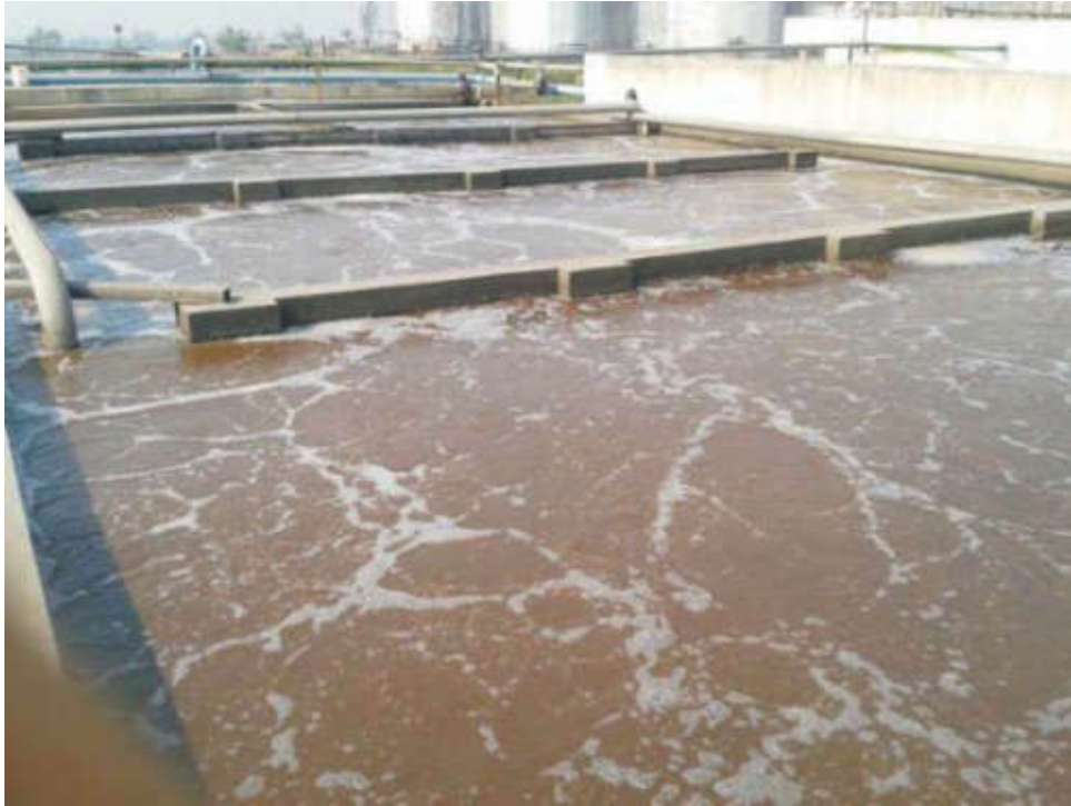
Old diffuse aeration tank
