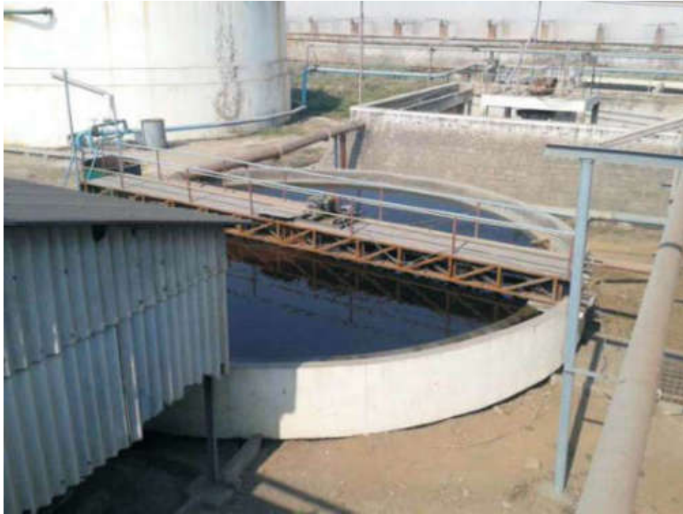
Secondary clarifier old stream
