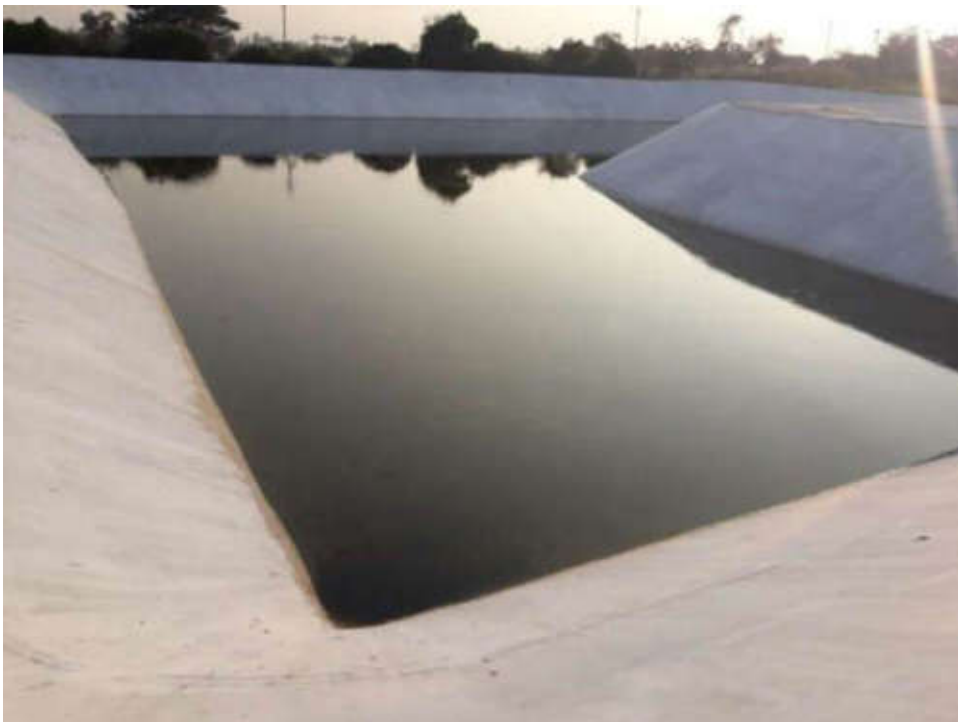
15 Days Storage Tank-2
