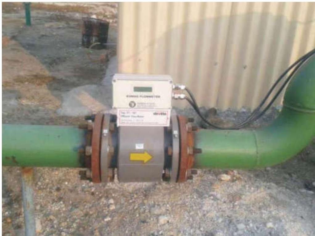
Flow meter for outlet Treated Water
