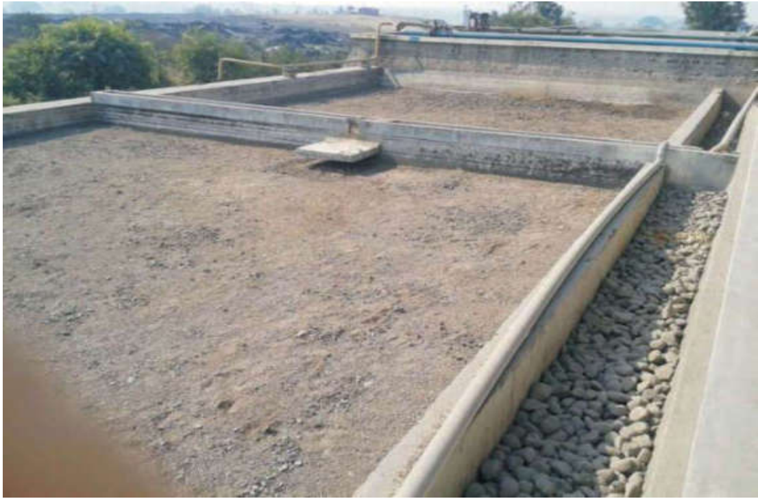
Sludge Drying Bed
