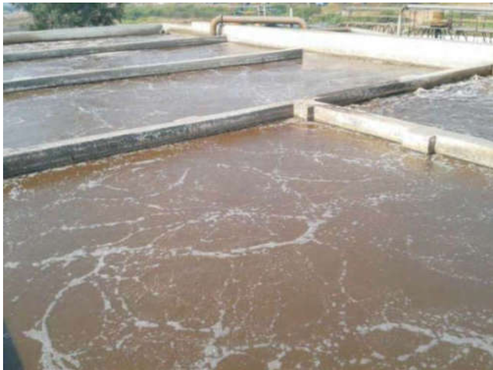
New diffuse aeration tank
