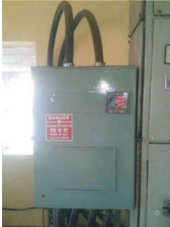
Electric energy meter for E.T.P.
